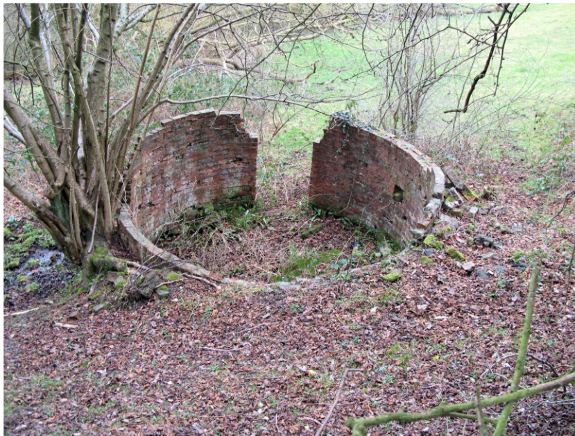
Figure 18. Circular building on the opposite side of Ironbridge Road – said to be an explosive magazine but may be associated with Coneybury Furnace. SJ 6815 0200. S. Dewhirst
