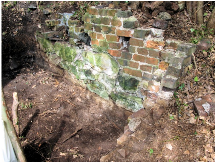
Figure 11. Building near engine house. Partial clearance of soil in 2008. SJ 6791 0785.
