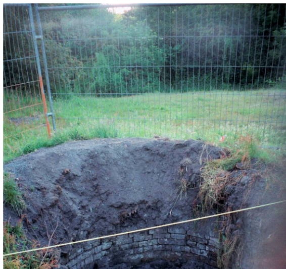
Figure 9 Haycop shaft in the 1990s. It had opened up presumably due to poor filling and was later capped by the Coal Authority. It is approximately 6'6" Diameter.
