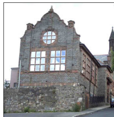
The only complete building now left on the Dowlais site, this library was built on land donated by Guest Keen and Nettlefolds Ltd. Its walls are faced with local stone and have red Alveley stone dressings from Shropshire, carved by T A Jones of Cardiff
