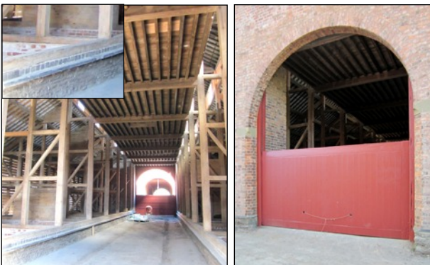
Below left, the inside of the barn with its 16 ft loft shows the remains of an old 8 ft gauge railway system. It also had a rat ledge both on the inside and the outside of the building (see inset). Below right, a close up of the newly restored portcullis at the other end of the building
