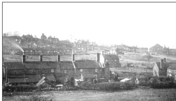
Some of the houses that were once owned by the Lilleshall Company and rented to their employees
