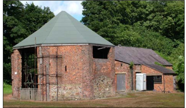
This octagonal building was probably the cannon foundry
