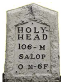
Telford's milestones along the Holyhead Road were stone pillars with recessed cast iron plates
