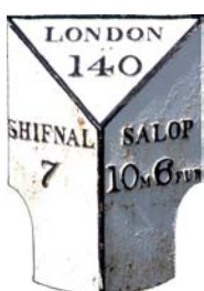
Telford's milestones along the Holyhead Road were stone pillars with recessed cast iron plates
