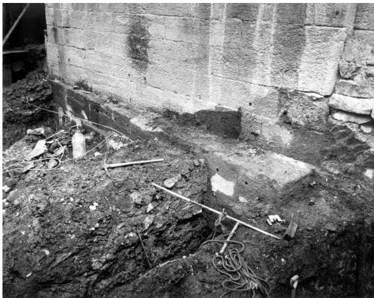
The original footings of the Iron Bridge were started out of line in 1777, seen here in 1974 prior to being buried under concrete.
