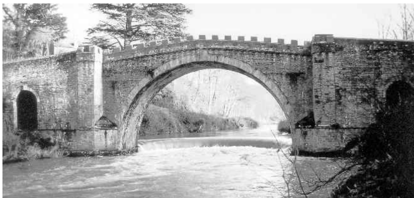
Pritchard's 50ft span bridge at Bringewood Forge, built 1772. Very similar to the shape used in the Iron Bridge.
