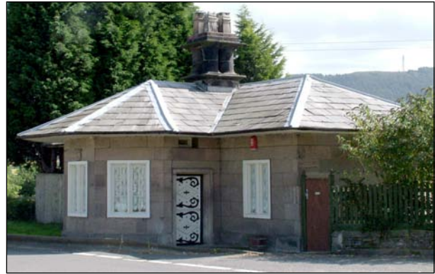
Toll houses were built throughout the country to control the traffic along the turnpikes. This one, which can still be seen on the A5 just west of Wellington, was one of those designed by Thomas Telford for his new Holyhead Road
