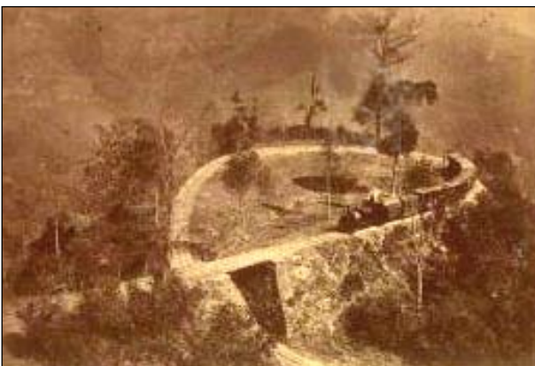
Agony Point on the Darjeeling railway has a minimum radius of 59 feet
