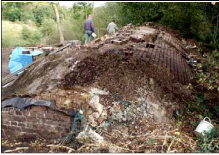
The old Down Well, now restored, was once Broseley's main source of water
