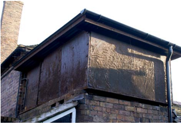
The cast iron water tank at The Lawns in Broseley
