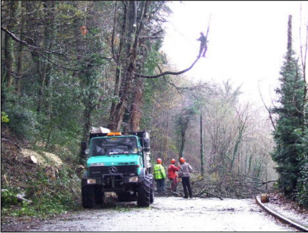
Work being undertaken in Ladywood was a major part of the Trust's 2005/6 Tree Safety Programme
