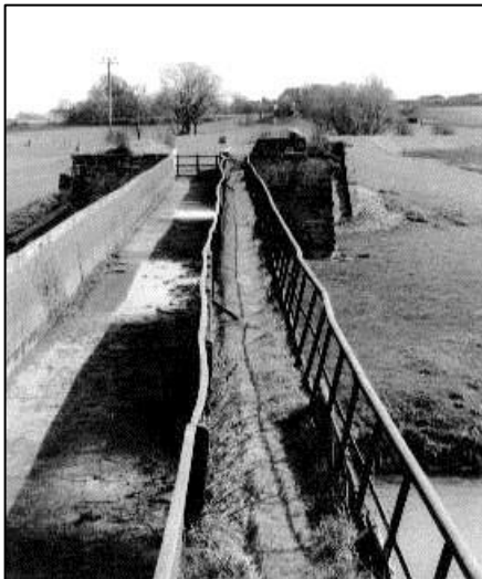
Telford's cast iron aqueduct carrying the Shropshire Canal over the river Tern at Longden. The aqueduct opened in 1797 replacing an earlier stone structure that was swept away by floods in 1795
