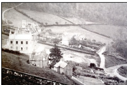
Coalbrookdale Literary & Scientific Institution under construction
