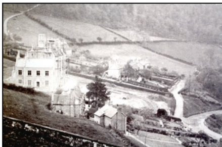
Coalbrookdale Literary & Scientific Institution under construction
