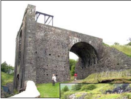
*The balance tower was used to hoist the wagons to the upper level*
