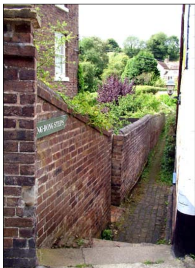
One of Broseley Wood's jitties, the Ding Dong Steps were so named after the ringing noise made by the soles of the boots worn by local workers
