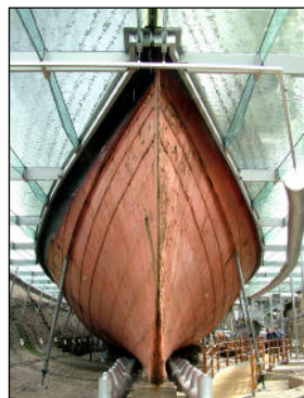
A glass ceiling at water level allows for a controlled environment to minimise corrosion
