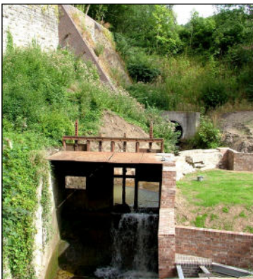
The Upper Forge Sluices are being restored and stabilised
